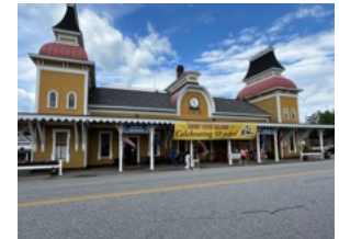
North Conway Station
